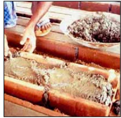
*Composite lintels and beams*
